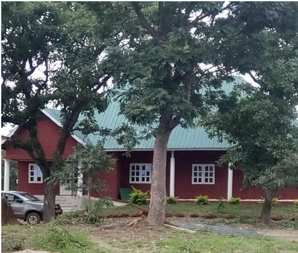
House in Natitingou
